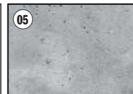
05 Station Viaduct Piers Concrete
