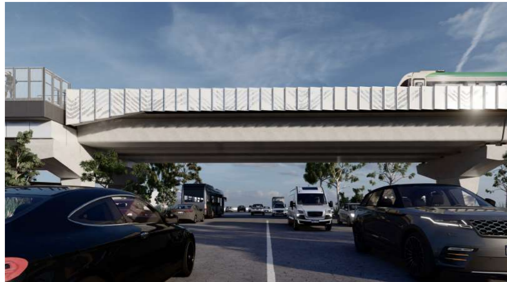
Interface at Station
