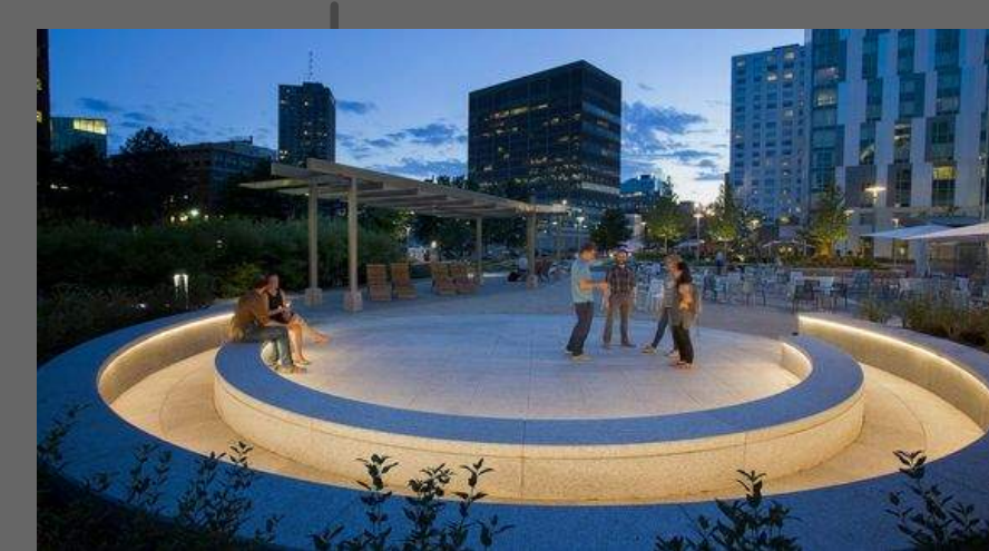
CIRCULAR SEAT ILLUMINATED WITH FLEXIBLE OUTDOOR LED NEON UNDER TOP MOST LIP PROVIDING SCULPTURAL AMBIENT GLOW TO SEATING AREA
