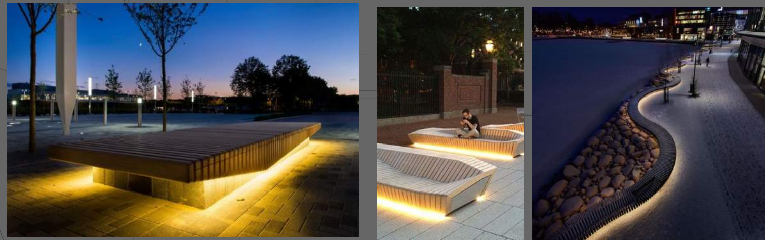
LIGHTING STRIPS INTERGRATED INTO SEVERAL SEATS. STRIP LOCATED IN EDGE SLOT BELOW TOP SLATS PROVIDES A SOFT GLOW SPILLING THROUGH GAPS AND INTO SURROUNDING SPACE.
