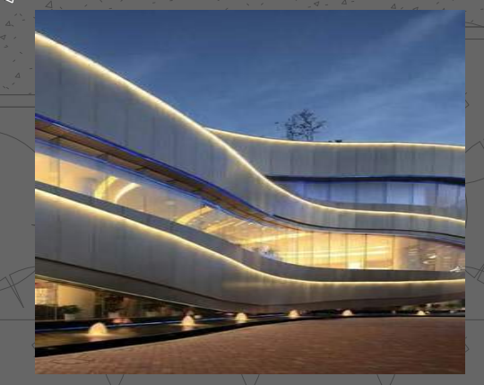
LED LINEAR PROVIDES LINE OF LIGHT AND GLOW DOWN THE FACADE OF THE STATION EXTERIOR WRAPPING AROUND EDGES UNTIL GLAZING COMMENCES
