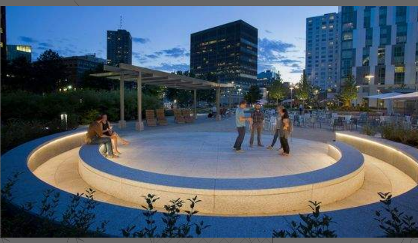
CIRCULAR SEAT ILLUMINATED WITH FLEXIBLE OUTDOOR LED NEON UNDER TOP MOST LIP PROVIDING SCULPTURAL AMBIENT GLOW TO SEATING AREA
