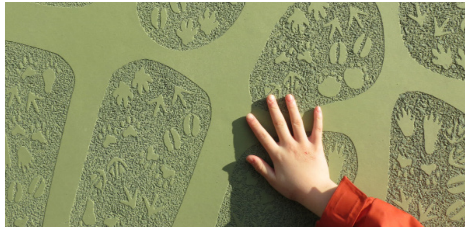
Tikkurila Daycare Graphic Concrete
