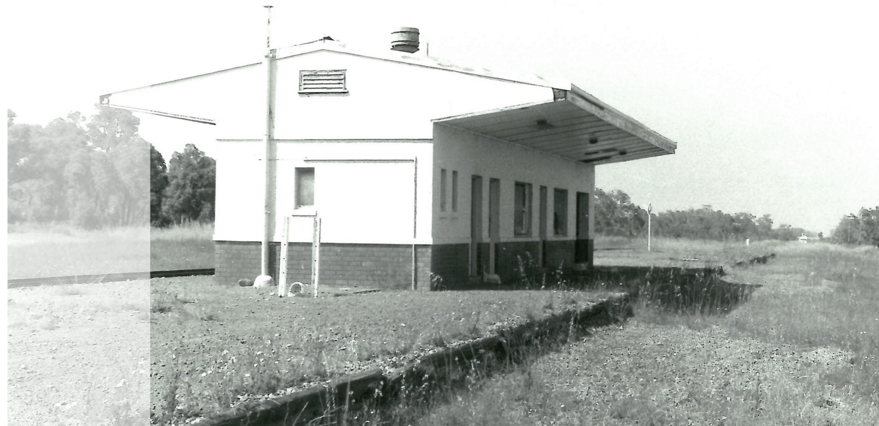
The old Byford railway station, shortly before demolition (1987). Photo: Ian L. Boersma
