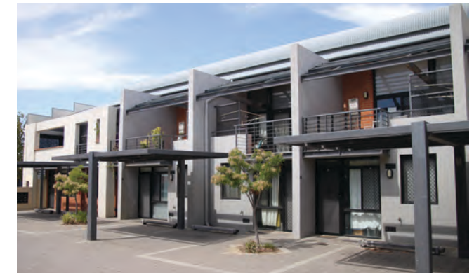
Photo G3.4d Providing a carport rather than a garage reduces the visual impact of vehicles on the street or communal area, is usually less expensive to construct, and can be located in the front setback area
