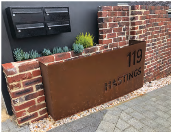
Photo G3.7a Water meters are screened from view behind this street address panel
