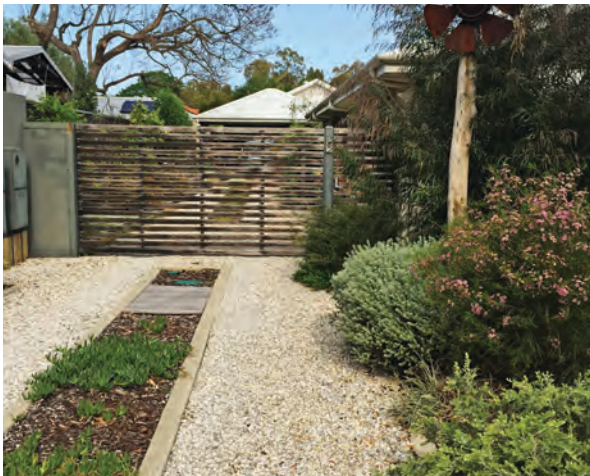
Photo G4.7a This shared driveway space has been designed and constructed to be fully permeable, and includes planted areas and a gravel surface
