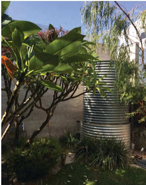
Photo G2.5a Compact rainwater tanks can be located within the primary garden area
