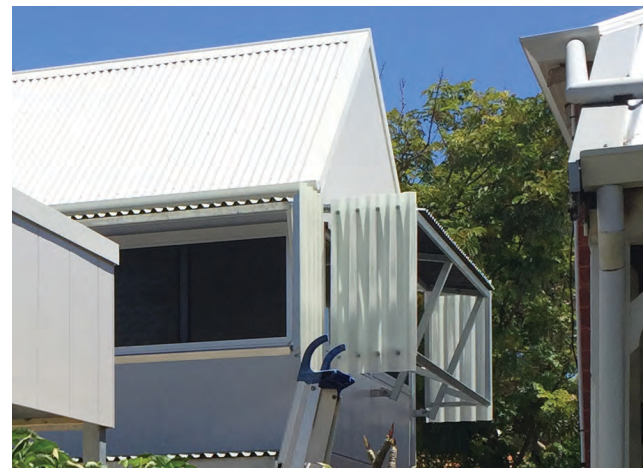
Photo G4.12c This window hood effectively restricts overlooking of the neighbouring property's rear garden without compromising amenity for the dwelling
