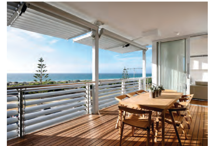
Photo G3.2a Adjustable louvres are an effective way to control sun, glare, privacy and ventilation through the day and year (PC)
