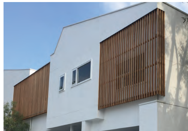
Photo G4.12b The privacy screening on this development has been effectively integrated into the building design
