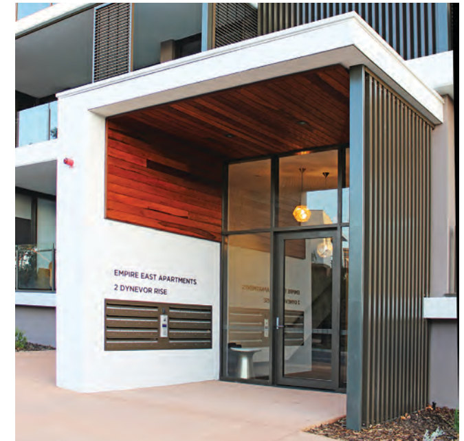
Photo G3.9a This development, designed for adaptability and universal access, has a well considered entry sequence with a wide, obstacle free path to the entry
