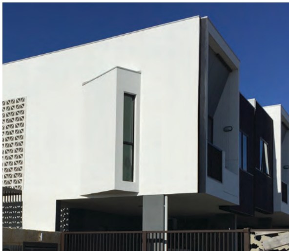
Photo G4.12a The upper level windows on this apartment have been oriented toward the communal space to help address visual privacy
