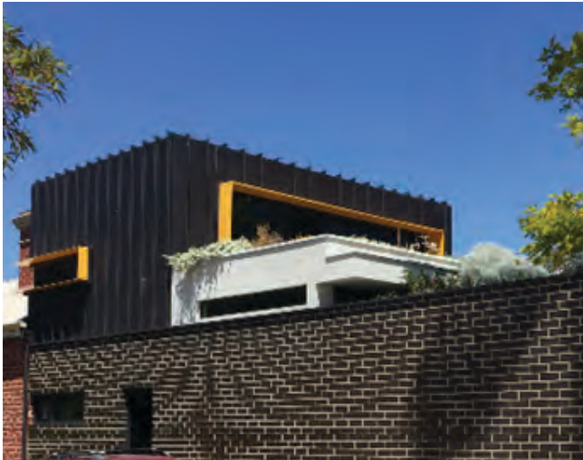
Photo G2.3c Planting on structure – a green roof on a rear addition to a terrace house
