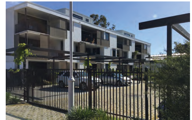
Photo G3.4b This secure communal parking area incorporates permeable paving and is co-located with other shared facilities, including community gardens and storage areas
