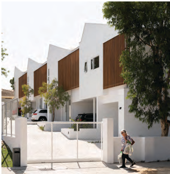
Photo G4.4a This row house development steps down with the slope of the site
