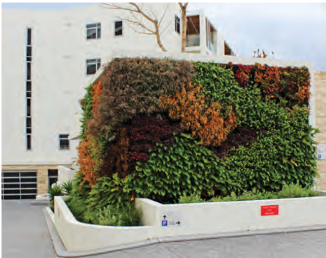
Photo G2.3b Planting on structure – a green wall at the entry to an apartment building
