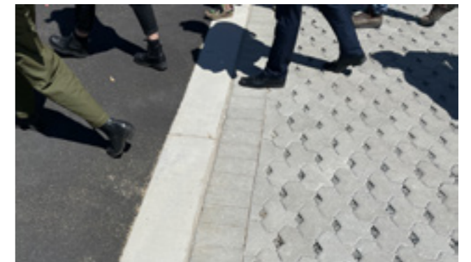
Bardi Lane, OneOneFive Hamilton Hill, Cockburn permeable paved parking bays around new trees
