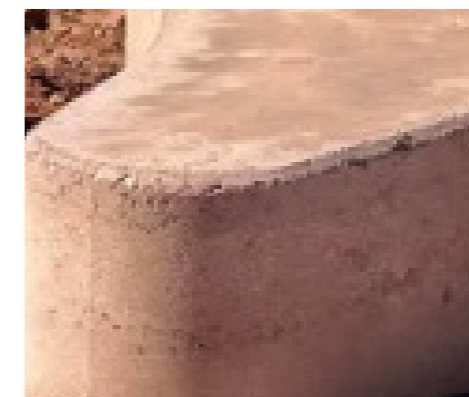
Coloured honed concrete (using recycled brick)
