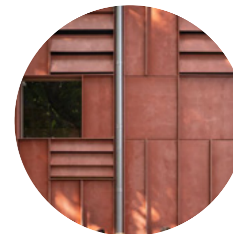
04 A SYSTEMATIC CONSTRUCTION
