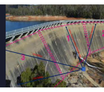
A compacted soil base of 8.7m x 8.5m would need to be established to accommodate the crane.
