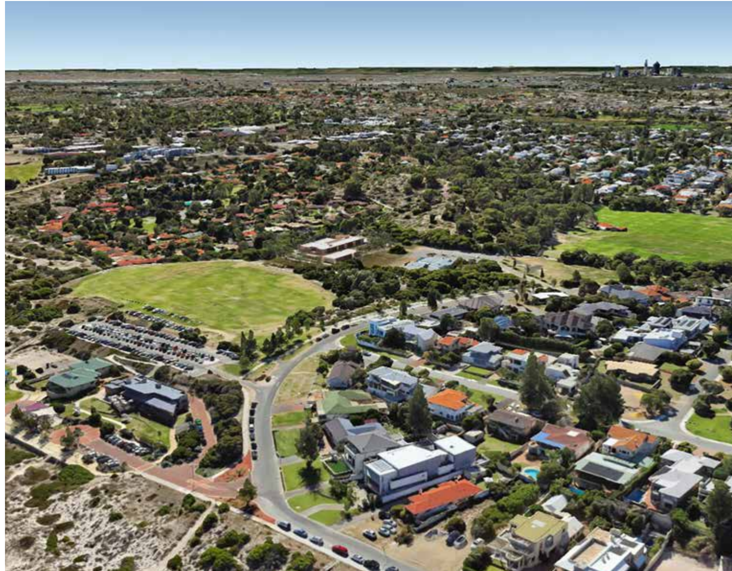
South-West Aerial View
