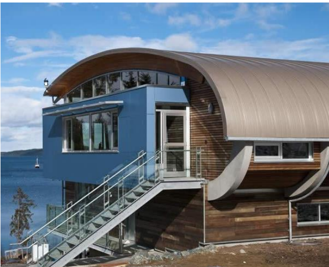
Deep Bay Field Station Building
