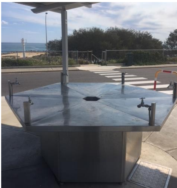
Fish Cleaning Station
