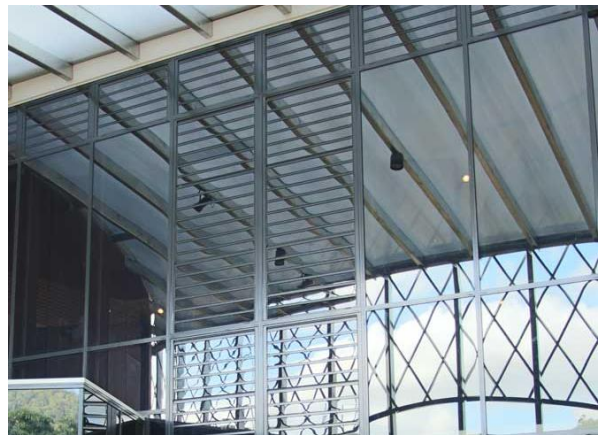
The Cairns Institute, Louvred windows
