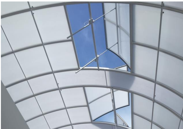
Barrel Vault Roof Lights
