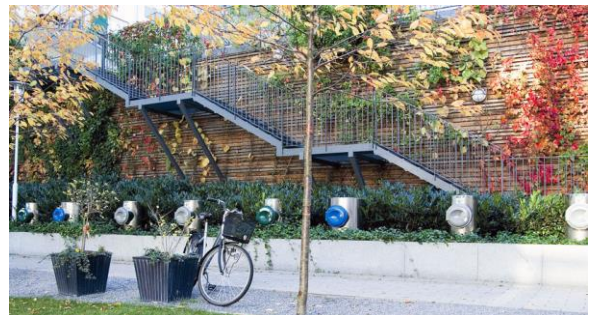
Waste Collection Integrated into Public Realm
