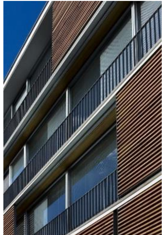
Mobile screens integrated to the building façade
