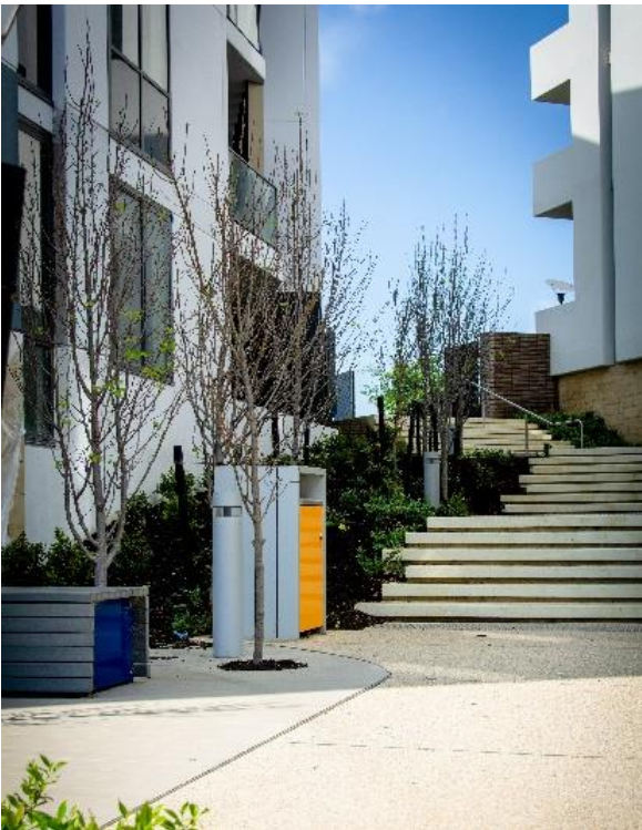
Utilities integrated within pedestrian accessways (Claremont on the Park, Australia)
