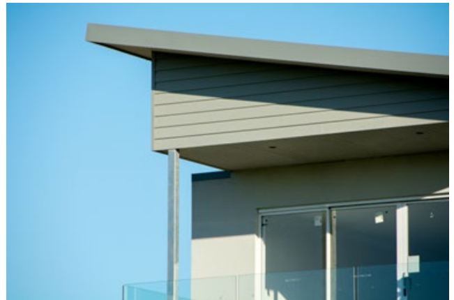
Image 14: Skillion roof form
