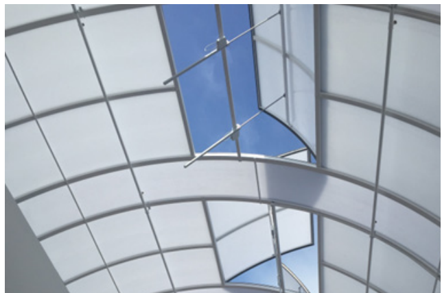
Image 13: Barrel Vault Roof Lights
