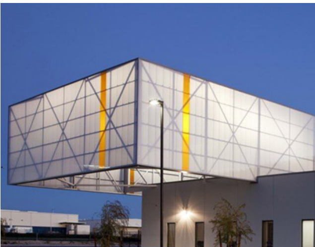
Image 31: Glass Box Illuminated Façade
