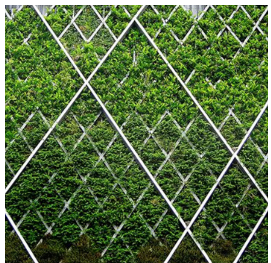
Image 20: Green Vertical Wall Screening Storage Structures
