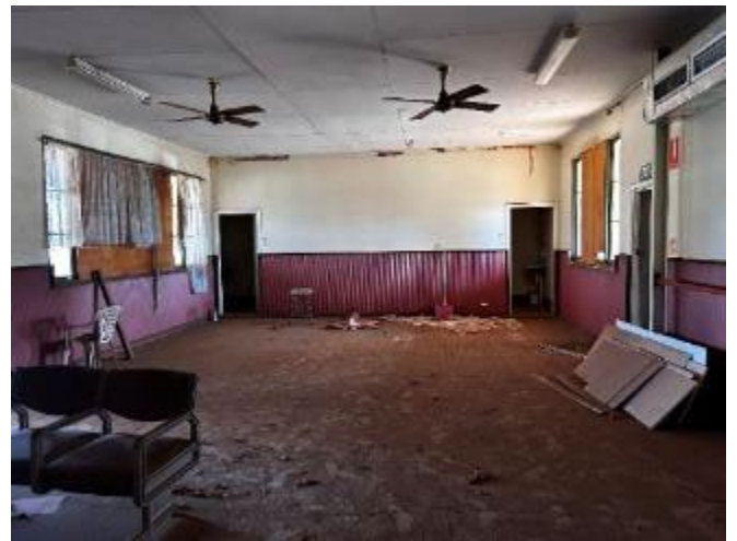
Figure 43: View through Main Hall No. 1 towards original section of school (Main Hall No. 2)
