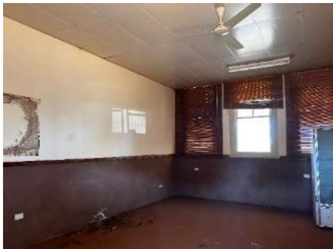
Figure 52: Original classroom (Main Hall No. 2)
