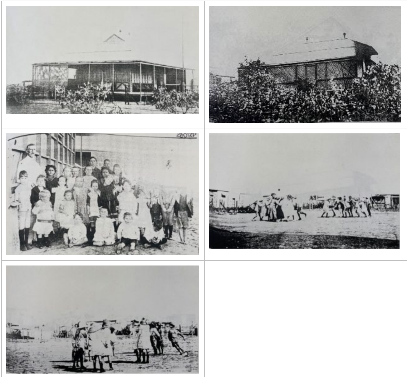
Figure 9 Views of Port Hedland School 1916. Courtesy SLWA Photographic Collection 28007P -28017P.
