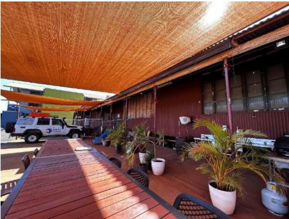
Figure 35: View along rear elevation
