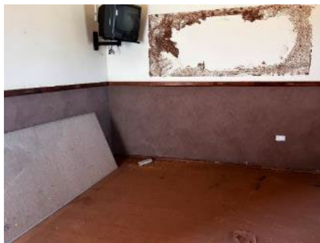
Figure 55: Dado around the walls of the original classroom
