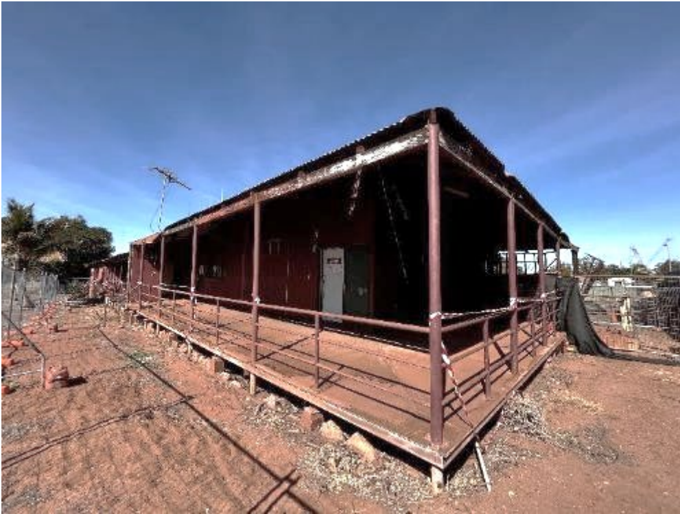
Figure 32: Original section of school at north western end
