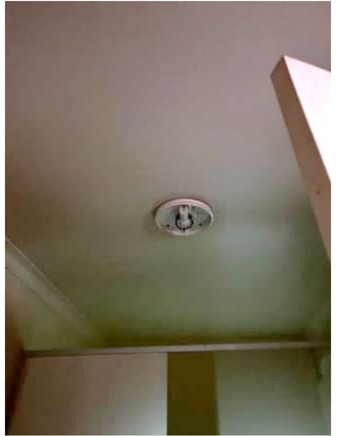
Figure 50: Plasterboard ceiling to toilet
