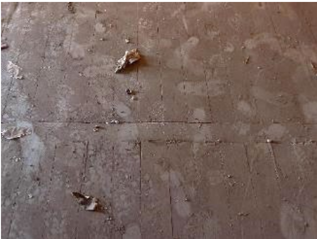
Figure 45: Timber floor Main Hall No. 1
