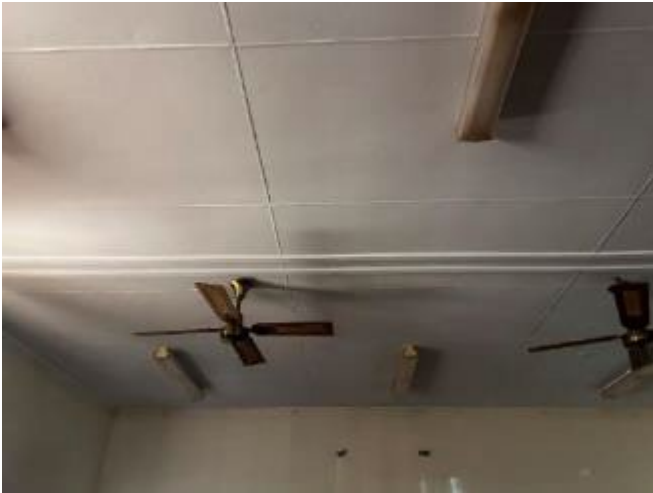
Figure 44: Ceiling in Main Hall No. 1
