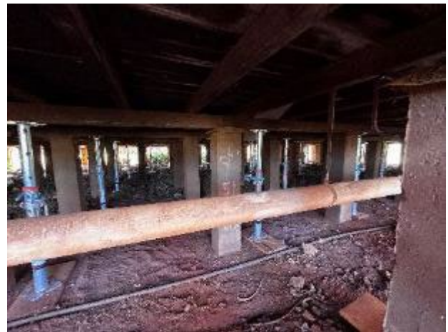
Figure 80: Acrow props underneath building
