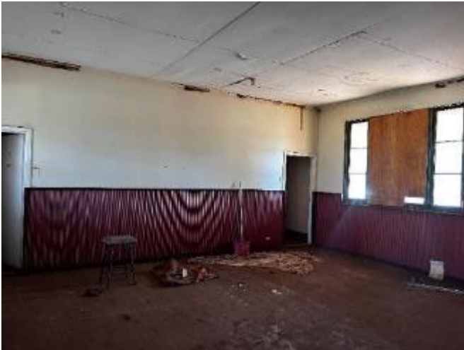
Figure 38: Main Hall No. 1 looking towards toilets
