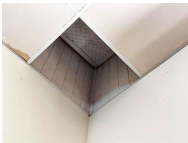
Figure 56: View through acoustic tile ceiling towards original level of ceiling
