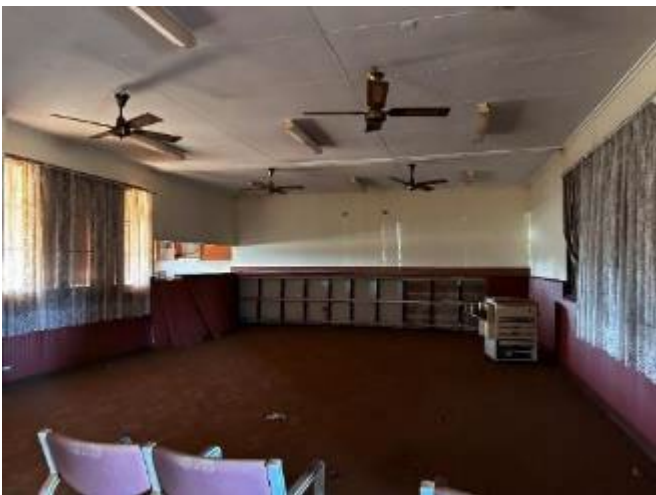
Figure 40: View through Main Hall No. 1
