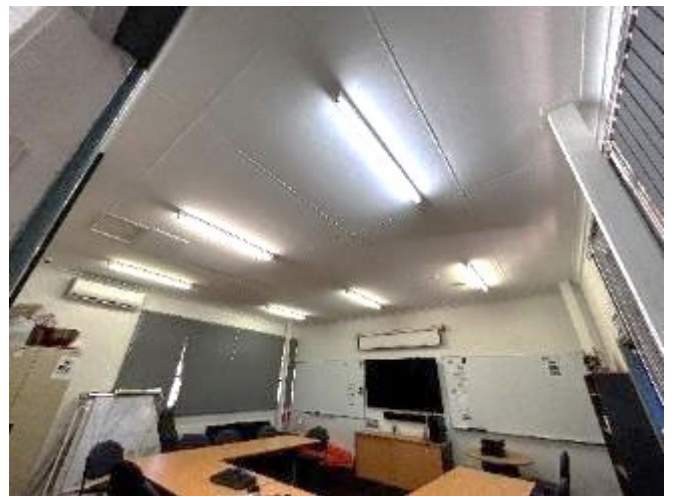
Figure 61: Ceiling to Meeting Room
