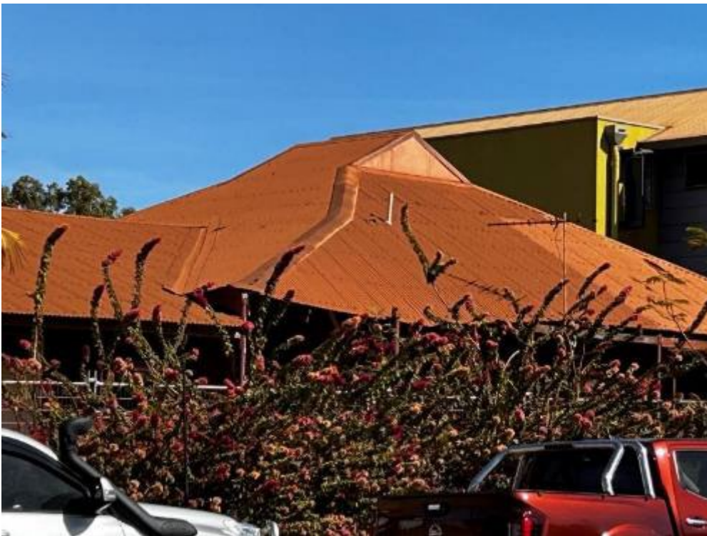
Figure 27: Sweeping hipped roof of original section of school
