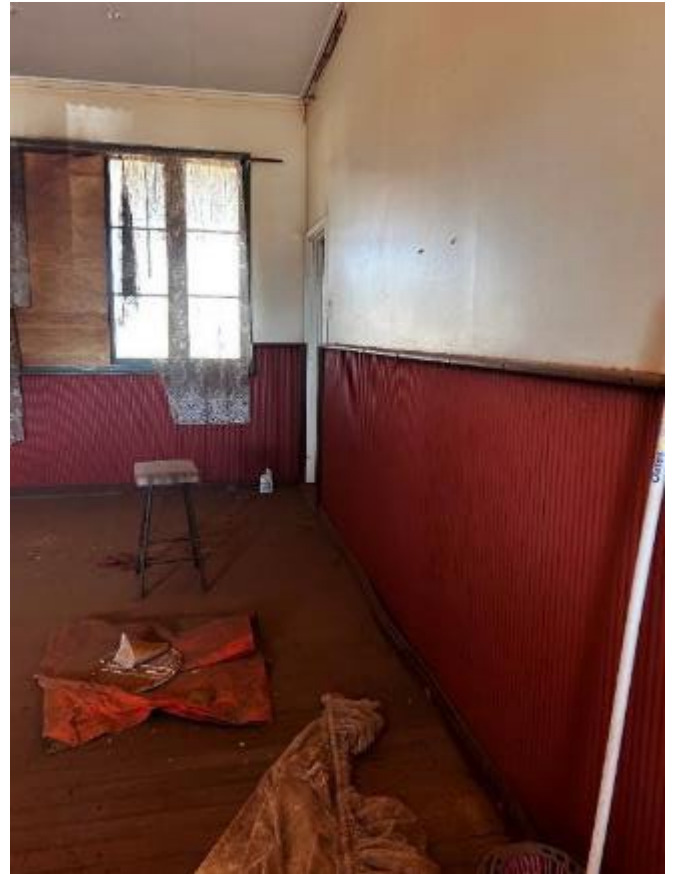
Figure 47: Custom orb dado along north-west wall of Main Hall No. 1
