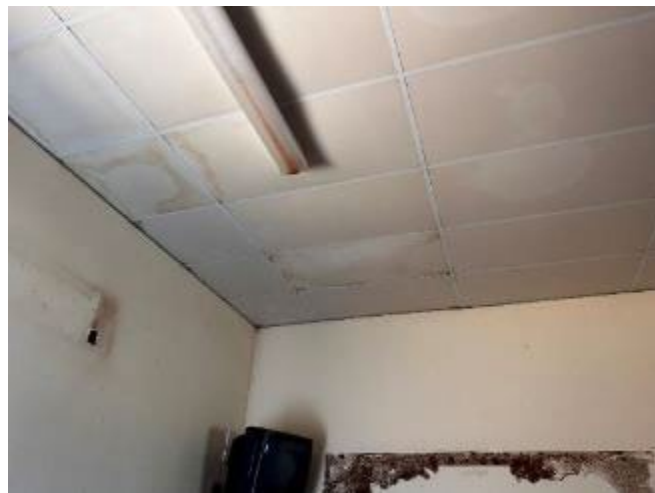
Figure 54: Acoustic tile ceiling
