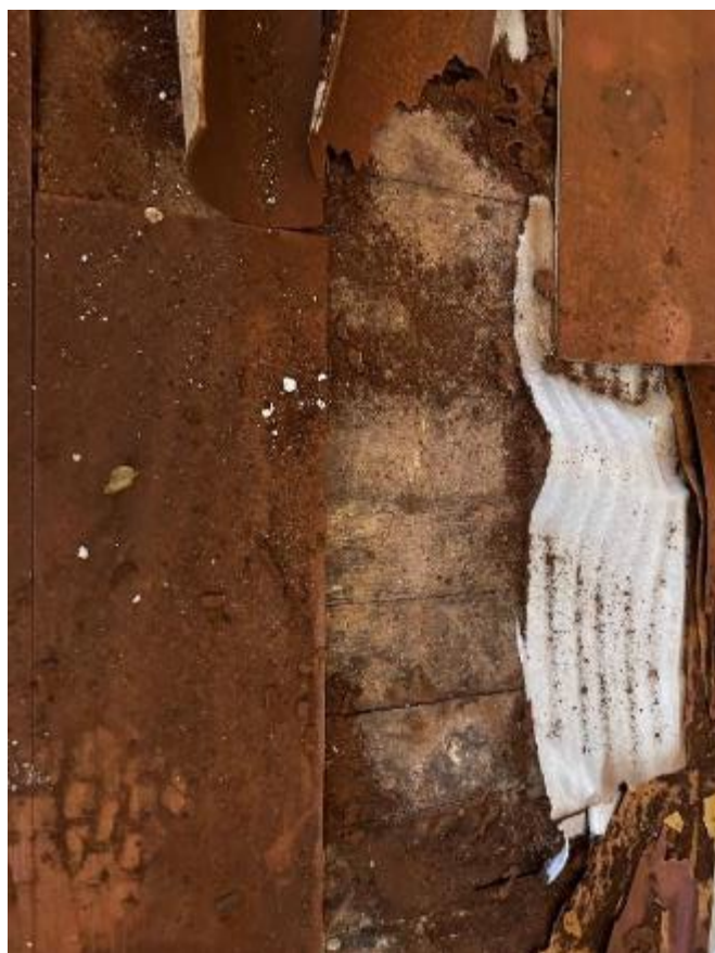
Figure 53: Timber floor under existing floor lining
