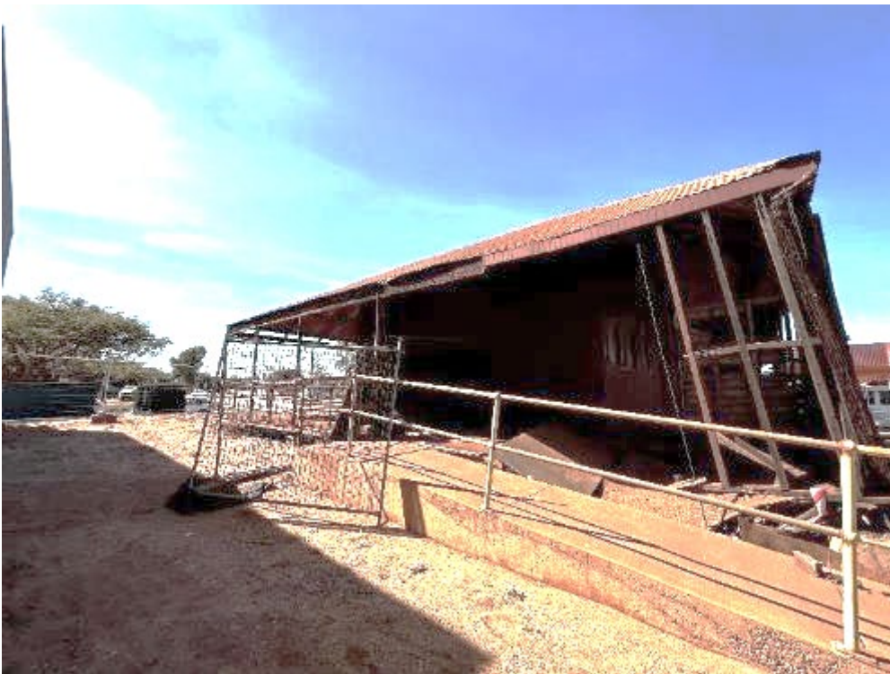
Figure 33: North west elevation – original section of school
