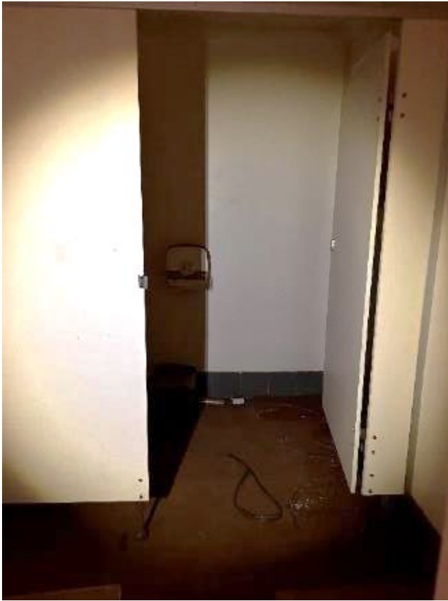
Figure 49: Typical toilet fitout
