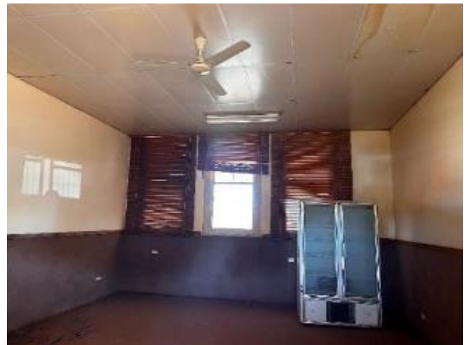
Figure 51: Original classroom (Main Hall No. 2)
