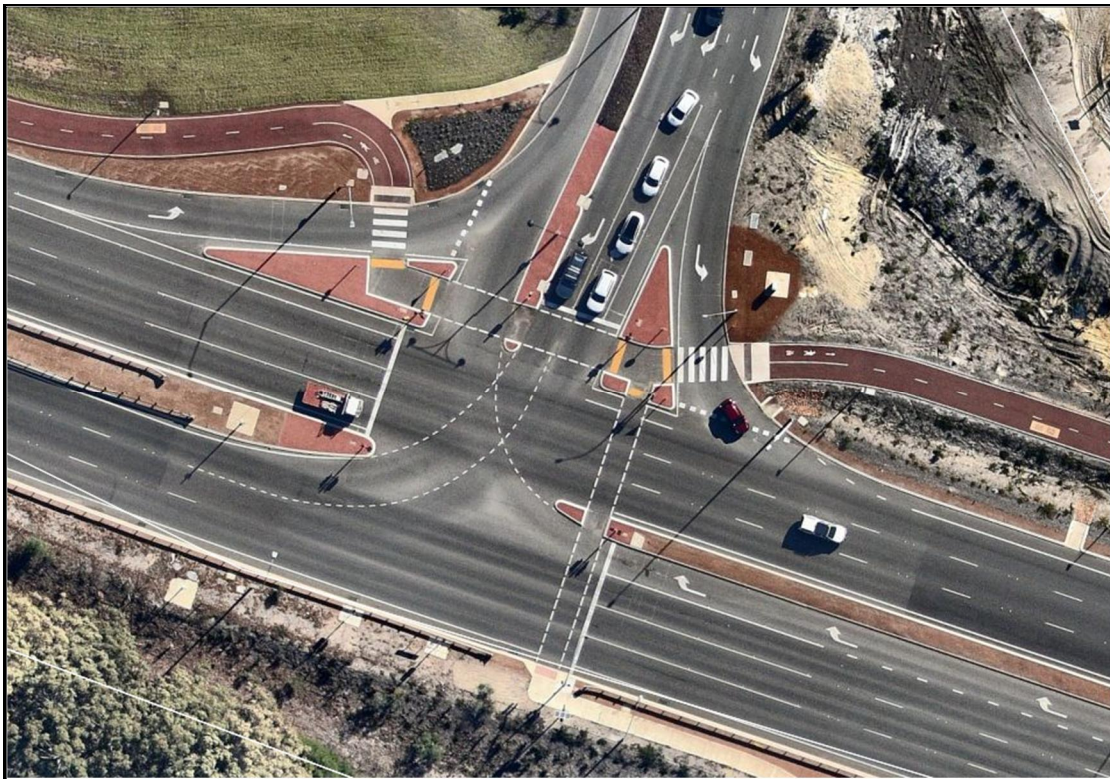
Figure 6 – Typical Intersection St Albans (Ghostgum Ave, Armadale Rd)
