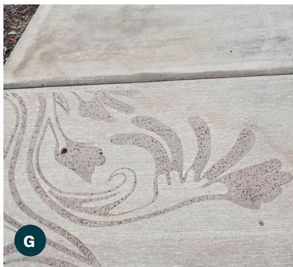
Broomed Concrete Footpath - Graphic Inlay
