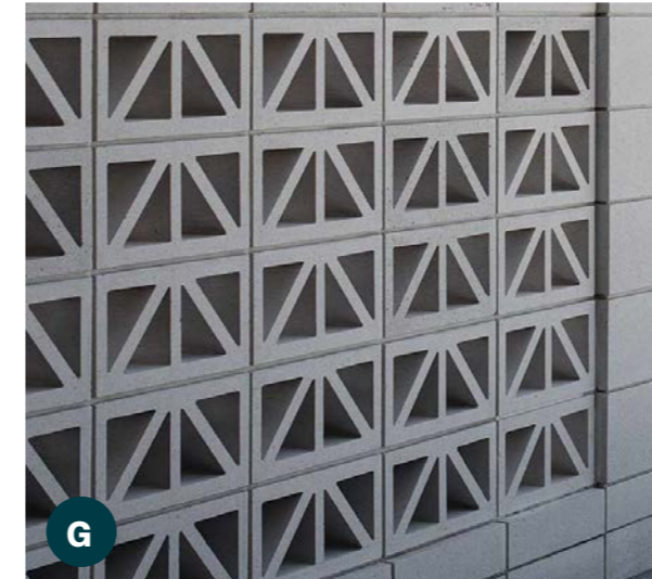
Fence Wall - Breeze Block (by architect)
