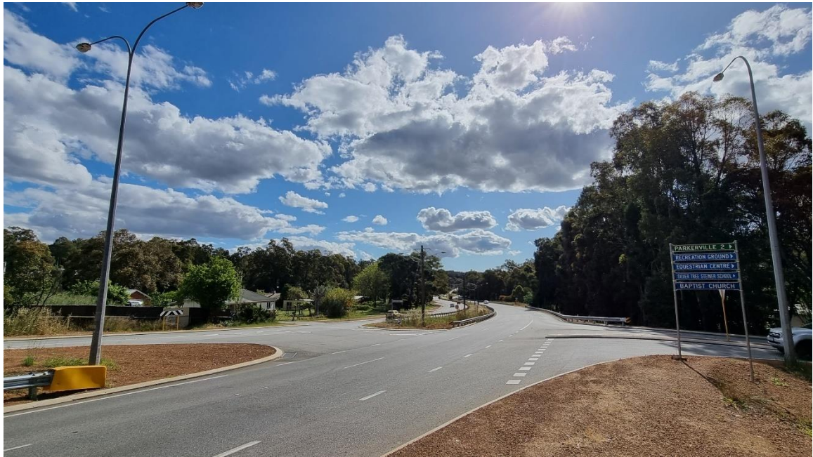
Figure 6: Great Eastern Highway/Seaborne Street Intersection
