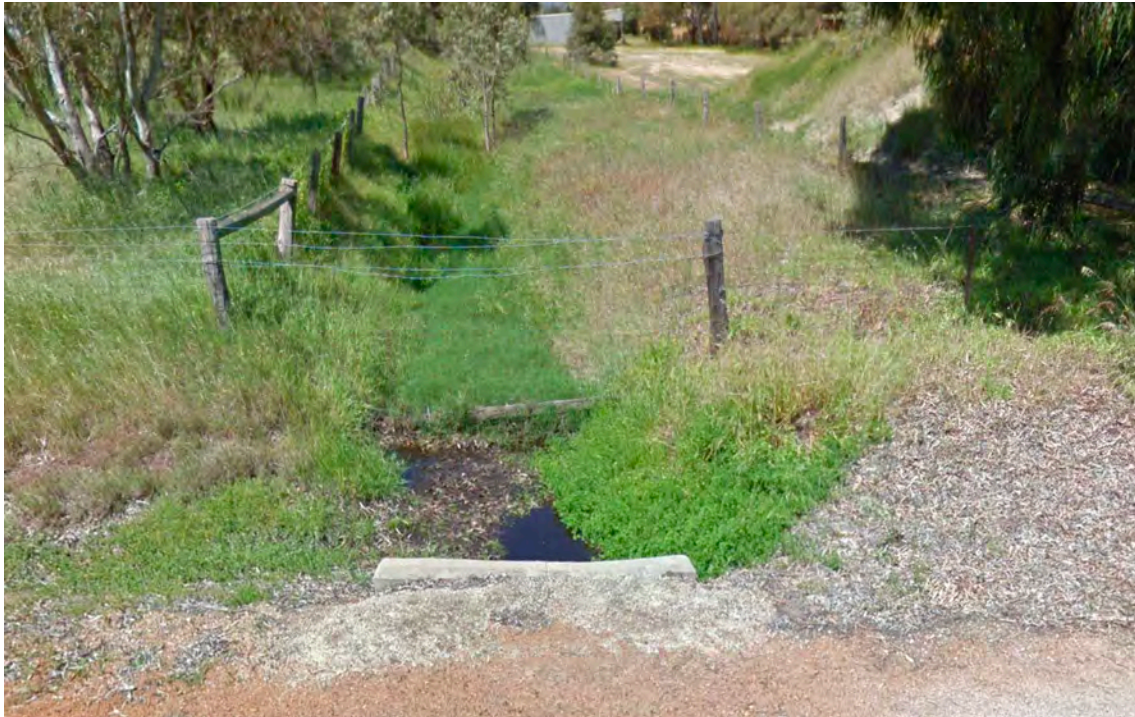
Figure 17: northern drain from Phillip Road (Google Earth)
