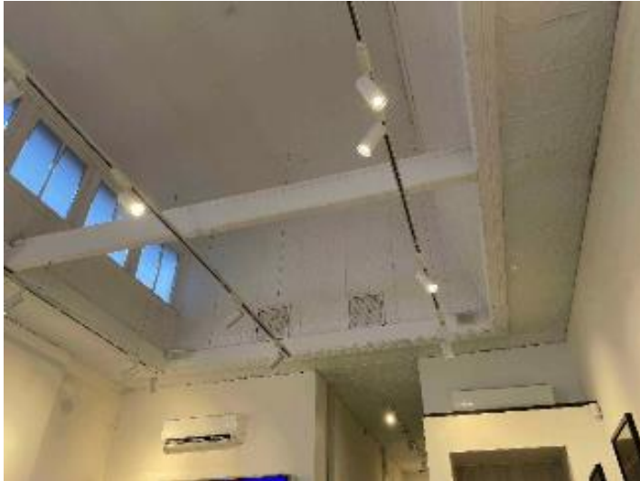
Figure 58. Internal View of No.296 Hannan Street
