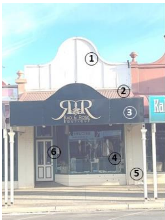
Figure 46. 288 Hannan Street detail
