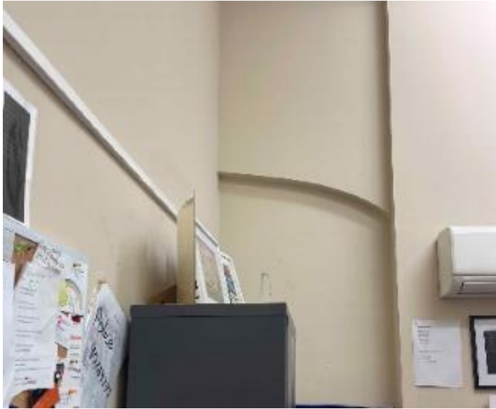
Figure 15. Internal View No.250-252 Hannan Street
