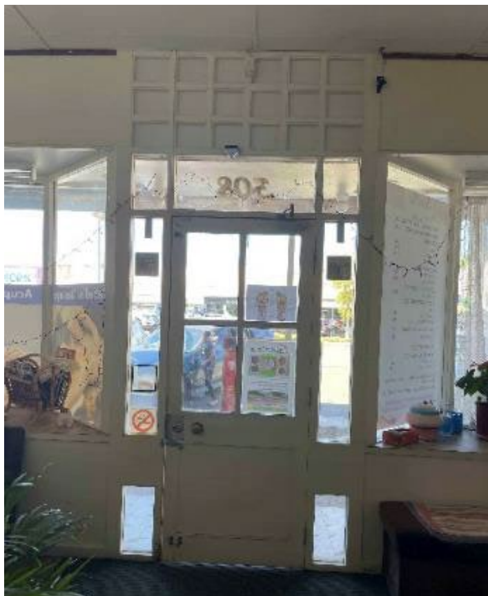
Figure 70. Internal View of No.308 Hannan Street
