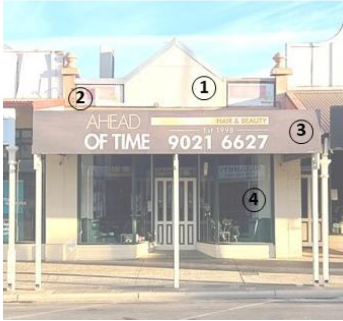
Figure 49. 290 Hannan Street detail
