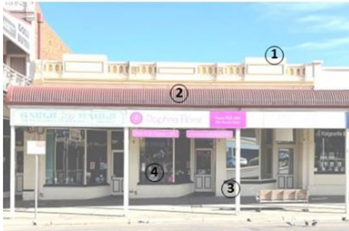
Figure 17. 254-258 Hannan Street detail
