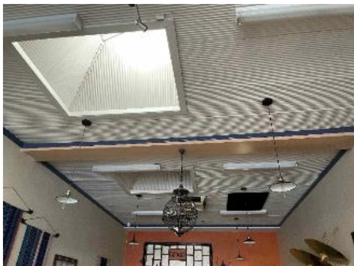
Figure 32. Internal View of No.268 Hannan Street
