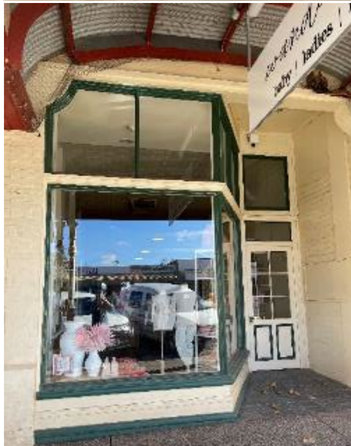
Figure 25. External View of No.262 Hannan Street
