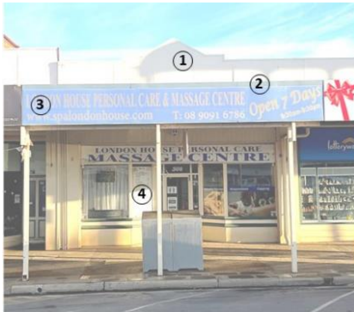
Figure 68. 308 Hannan Street detail
