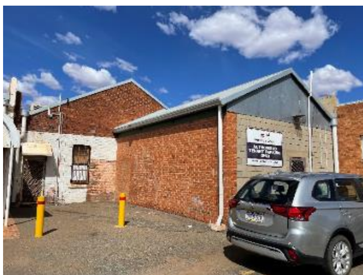
Figure 57. External View of No.294 Hannan Street
