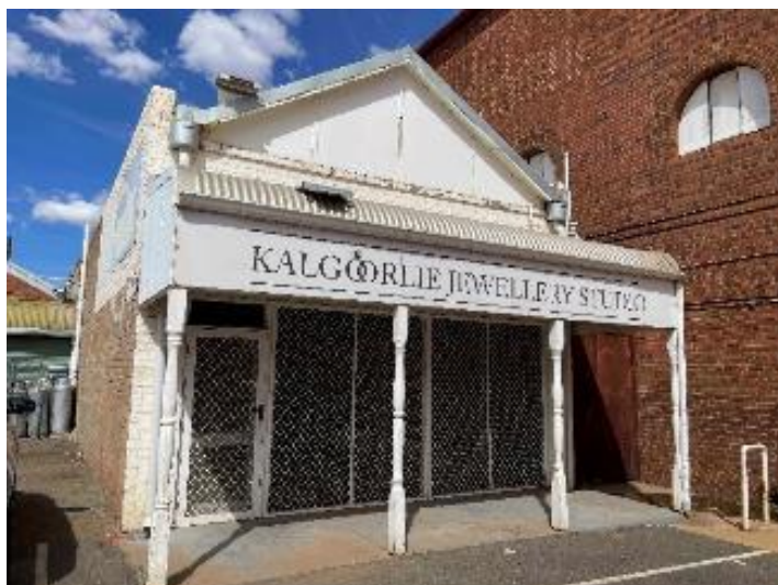
Figure 78. External View of No.260 Hannan Street
