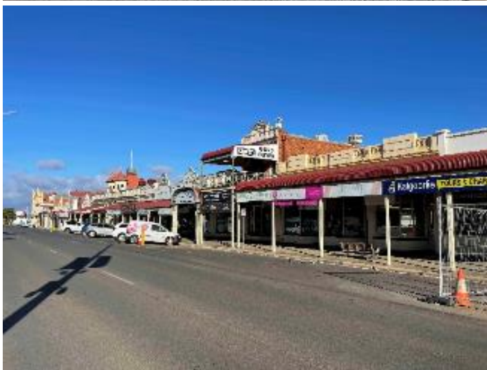
Figure 11. View looking west from 250-314 Hannan Street.
