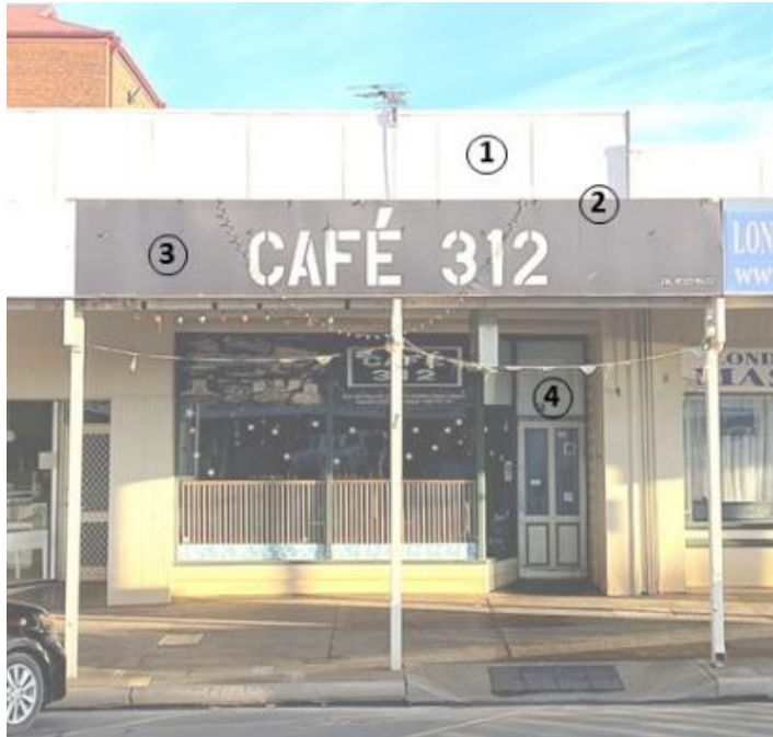
Figure 71. 312 Hannan Street detail
