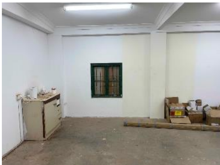
Figure 39. Internal View of No.272-280 Hannan Street, Former Sales Yards
