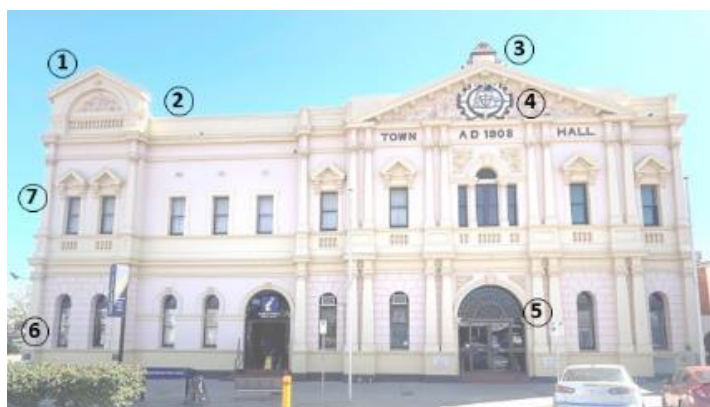
Figure 79. 316 Hannan Street detail
