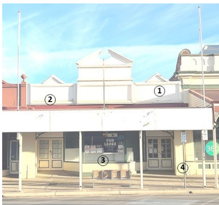
Figure 40. 282 - 284 Hannan Street detail
