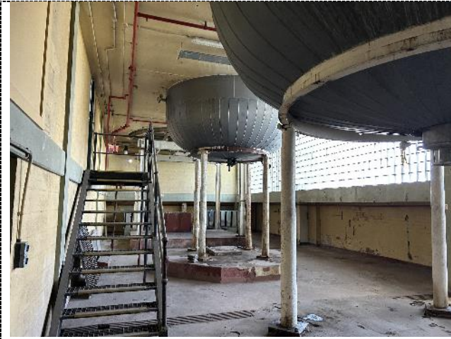
Figure 25. The underside of the brew chambers below the mezzanine floor.
