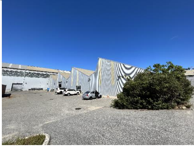
Figure 16. The saw tooth roof warehouse bays extend to the rear of the office section and were reduced in size in 2011. The distinctive roof form has been retained and the new east elevations have been clad with corrugated metal sheeting with two strips of translucent sheeting to each bay to allow for natural light. The southern plane of the roof form is glazed.
