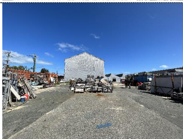
Figure 7. View looking west through Lot 220 towards the factory building with the remnant saw tooth roofed factory buildings in the background.
