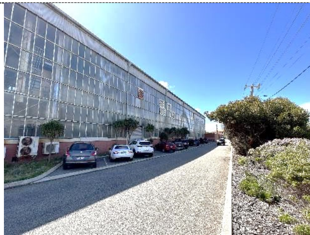
Figure 6. The southern side of the building is built hard to the boundary along Coventry Parade with angled parking along Coventry Parade.
