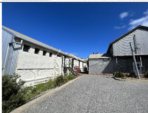
Figure 15. North elevation with two storey detached 1995 Administration Building addition to the north, and parking area created as a result of the demolition of a c.1940s workshop. The north elevation presents in a single storey form with white painted brick finish. Windows are a mix of larger office windows with horizontal louvers and high level metal framed openings. This elevation does not contain any distinctive features.
