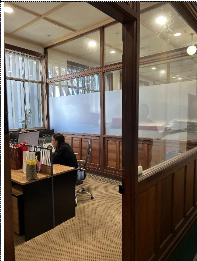
Figure 21. Typical office formed by timber and glazed partitioning. The partitions throughout the northern office area are a mix of original and altered. Changes to the details in the timber partitioning is evident in places, for example widths of timber panels and details on the architraves indicate that new material has been introduced and original fabric also altered to suit occupier requirements.
