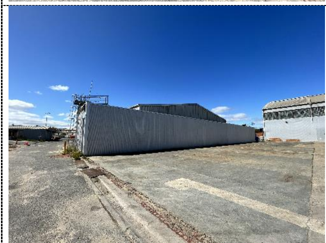
Figure 9. Recent shed structure which sits alongside the eastern curtilage boundary.
