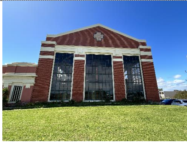
Figure 10. The large volume factory section has a classical presentation at the front elevation, with a classical balance of horizontal banding and vertical brick pilasters formed by the recessed vertical glazed panels under a gabled roof line.
