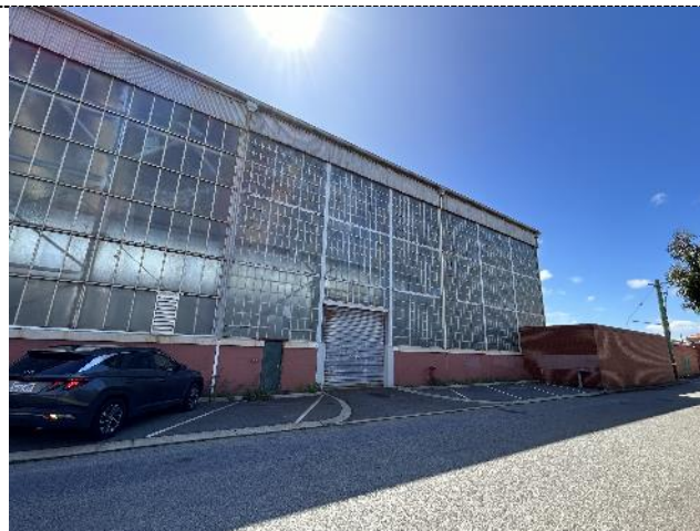
Figure 14. Contrast of glazing styles in the south elevation. The majority of the glazing panels are large rectangular panels with metal glazing bars. The last two bays at the eastern end have much smaller panes which are consistent with early photographs of the place, and of the 1947 expansion. The glass panels are set on a brick plinth with a rendered band separating the brick from the glazing panels.
